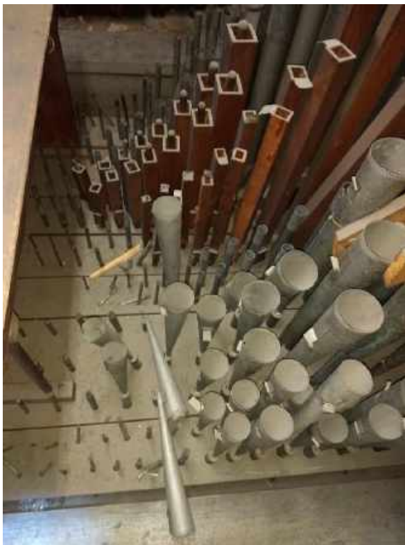
IN THE GREAT DIVISION, PIPES ARE KNOCKED OVER AND SOME APPEAR TO HAVE BEEN STEPPED ON.
